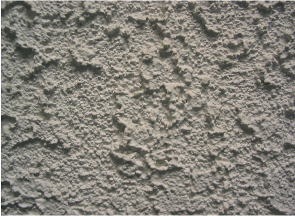
Figure 5: Example of stucco surface.
