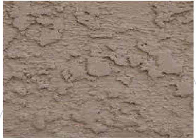
Figure 6: Example of troweled surface.
