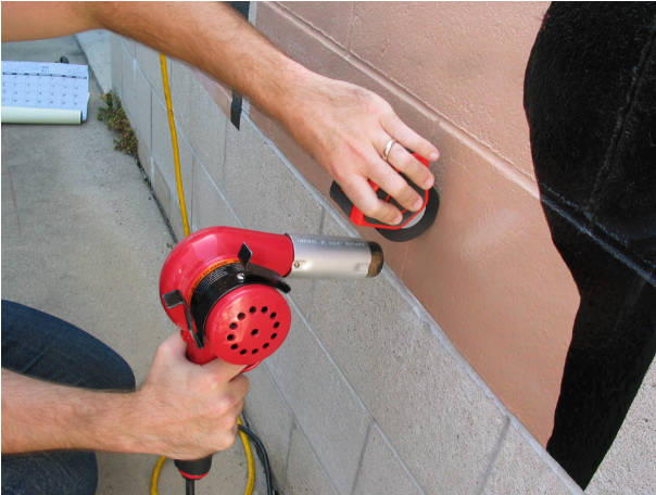
Figure 1: Installing vertical grout.
